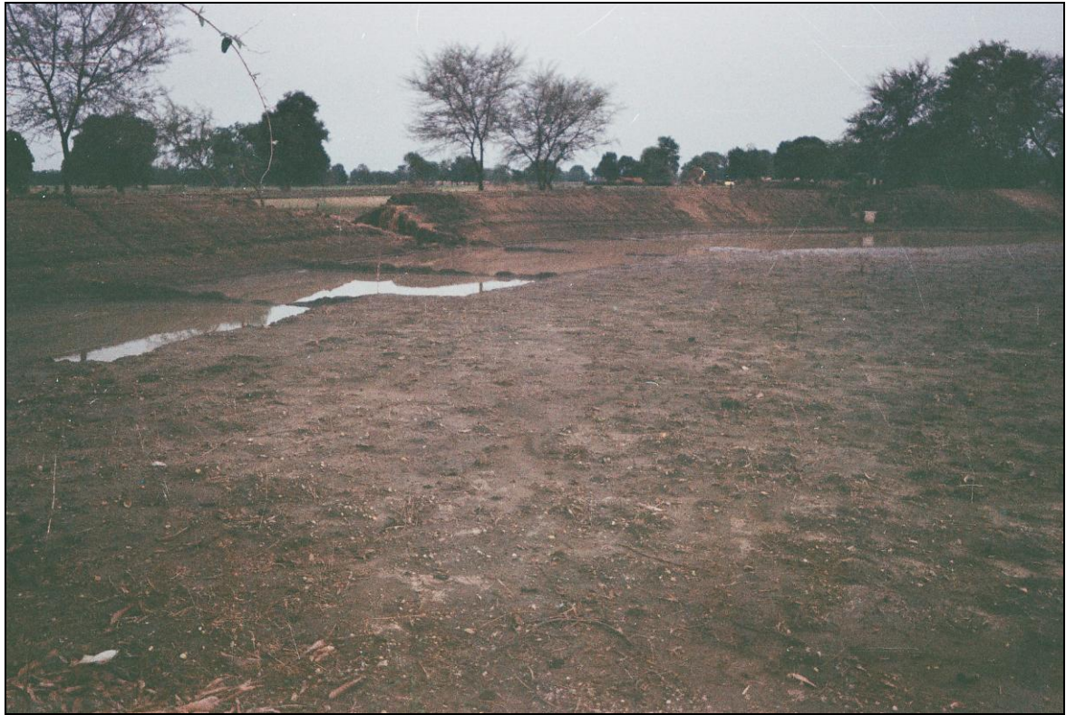
PLATE 3: A BUND DAMAGED DUE TO HEAVY RAINS
