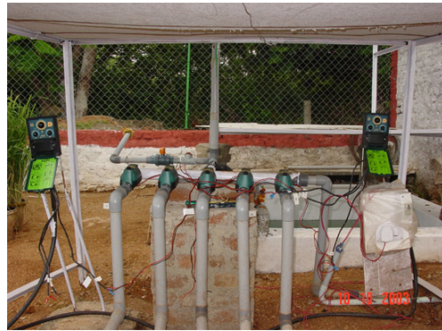
Fig 10b: Digital irrigation controls used for regulating water supply to different plots
