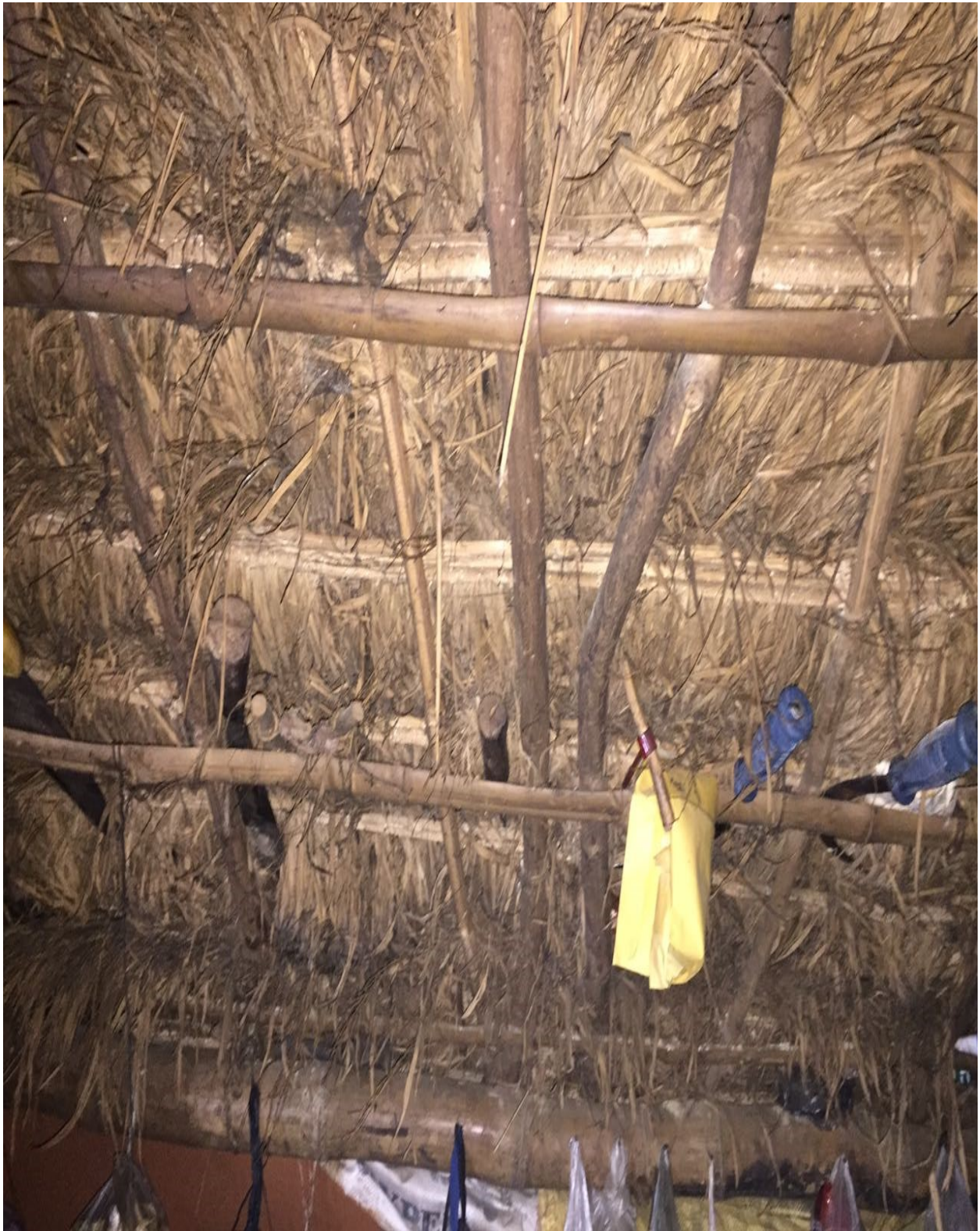
Figure 3.5. Roof of a traditional Saura House
