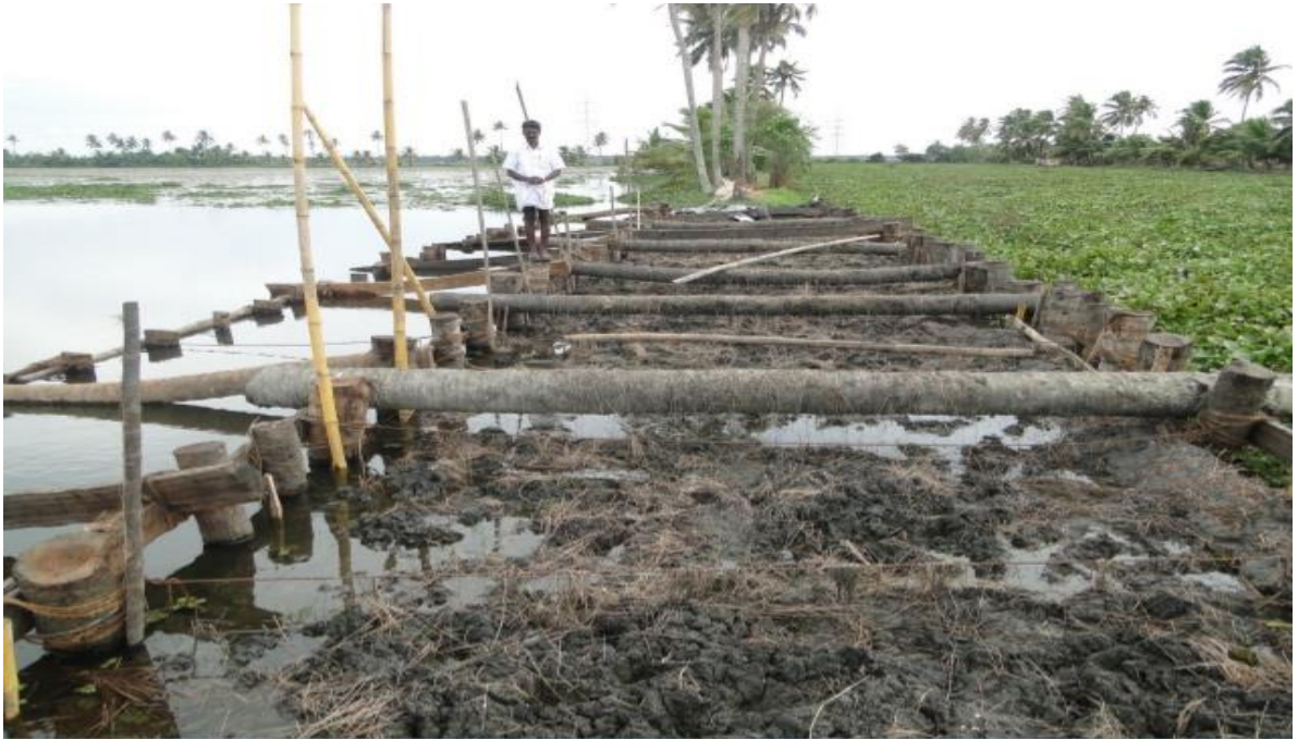
Photo 3.1: Construction of Bunds with natural material
