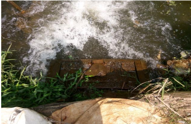
Photo 4.3: Water drawing out from field to the canal through Iron sluice of pette-paara
