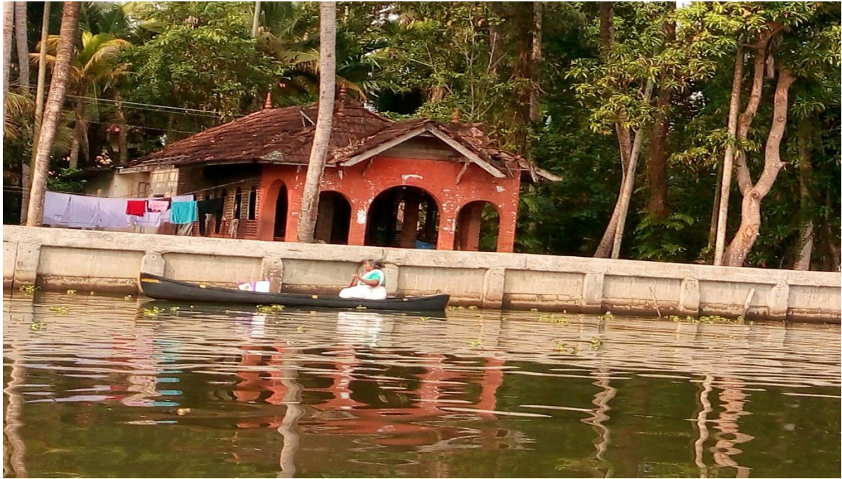
Concrete bunds in Kuttanad region
