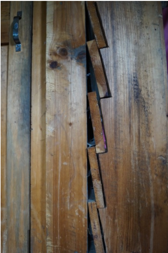
Image 12 (Left): Interlocked wooden planks in the walls of a typical Memba house
