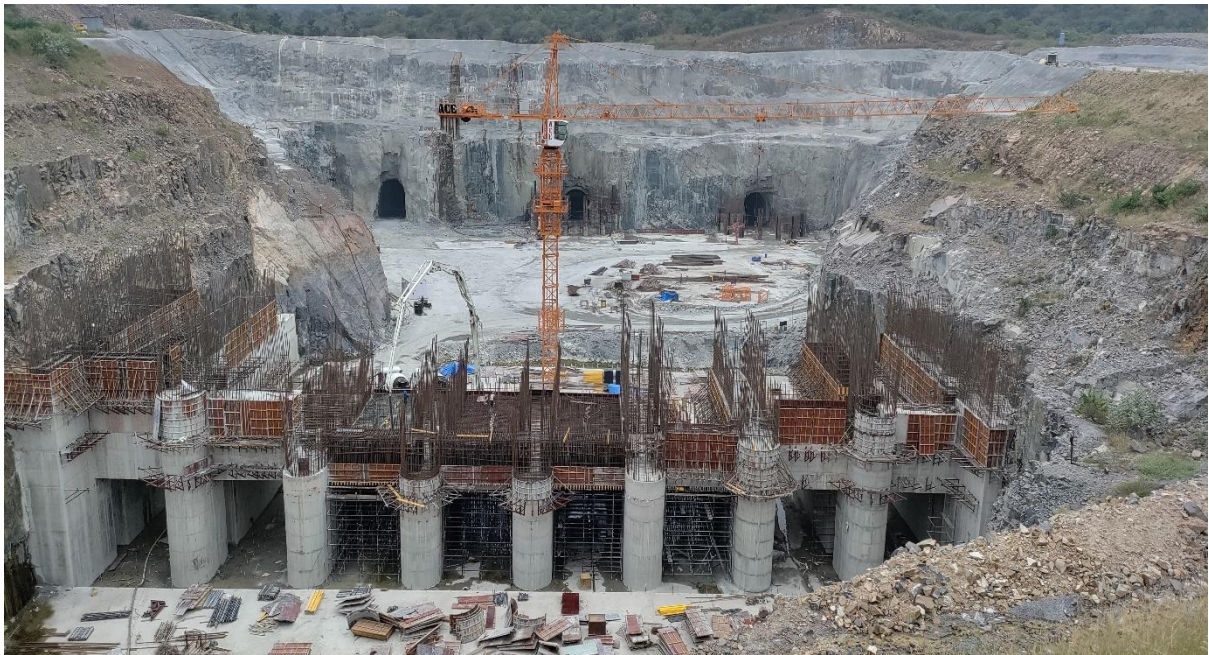
Frame No.2 Lift Irrigation Starting Point
