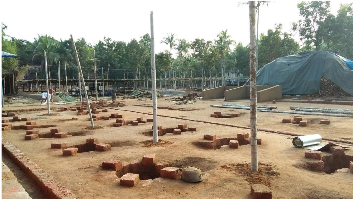
Photo 4.1: Construction of hearths in kitchen and dining area at Karivellur Muchilottu
