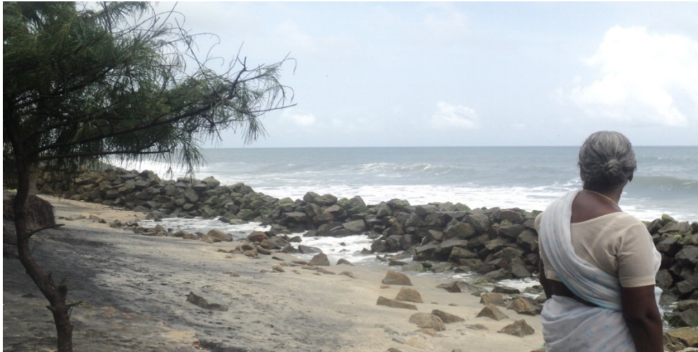
Image 4.1: Overtopping in Alappad Panchayat
