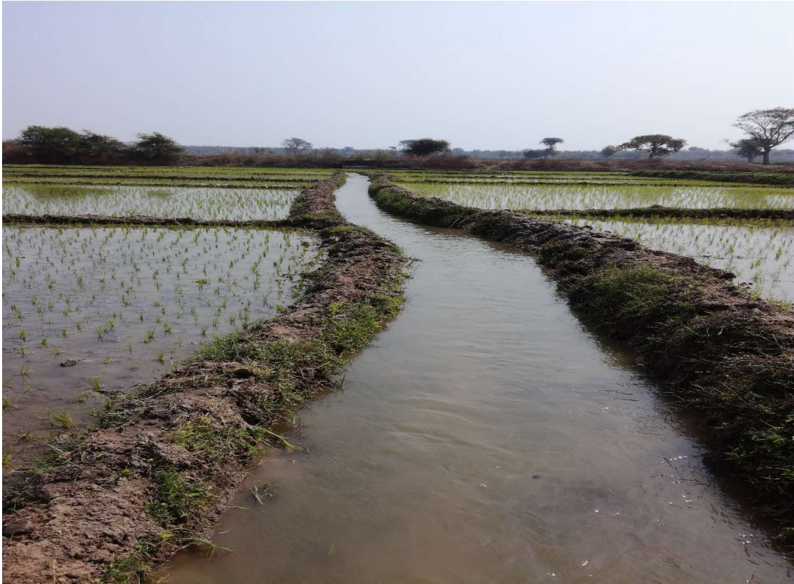
Figure 12: Canal traversing the fields
