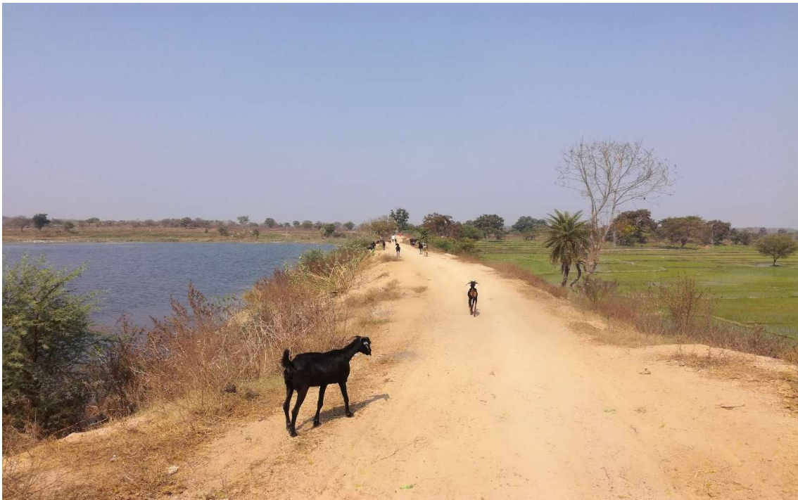
Figure 2: Village Tank Bund and adjacent fields.
