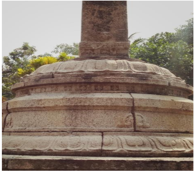
Fig.20. Base of the Niranam Open Air Cross
