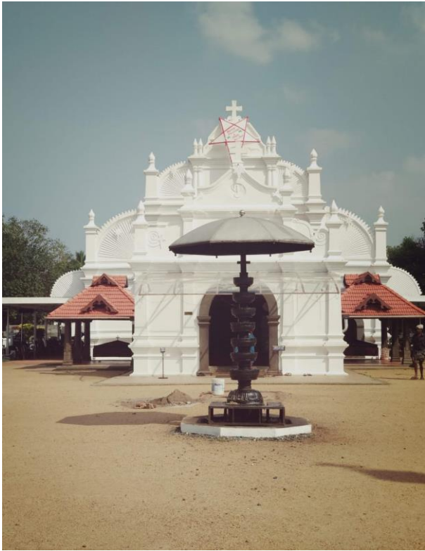
Fig.7. Front view of St George Orthodox Church Paliekara
