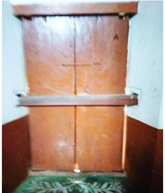
Fig.28. Door locking system, St Xavier's Church, Velur
