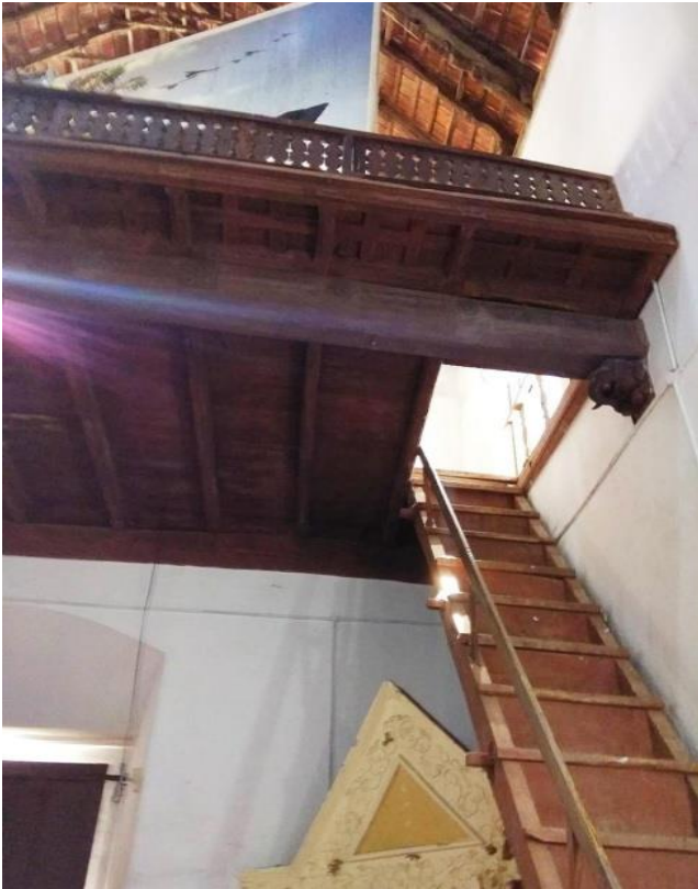
Fig.27. The stairs leading to the balcony at the Western end of the Hykala at Udayamperoor church
