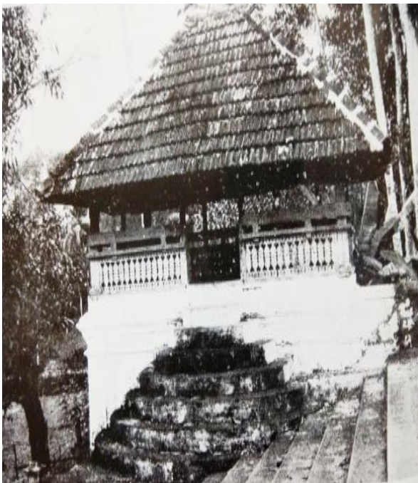
Fig.13. Kottupura or Vadyapura, Palai Cathedral
