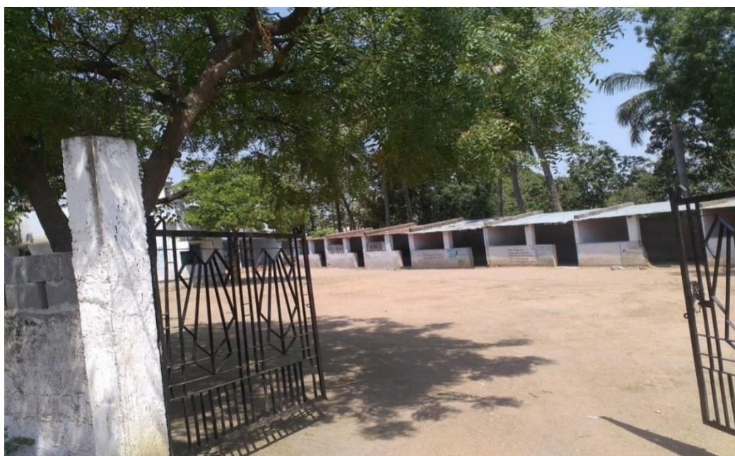
Picture No. 6.4 Rented Semi-pucca school building of Navabharathi High School, April 2015
