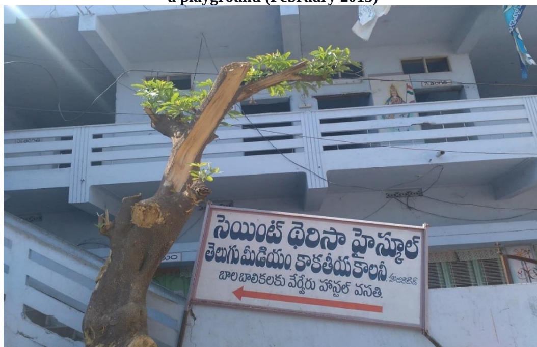
Picture No. 4. 5 Rented school building of St. Theresa High School (TM) without a playground (February 2015)
