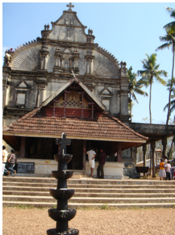
Fig.1.The Entrance Porch of the Church of Kadamattom (Image Source:
