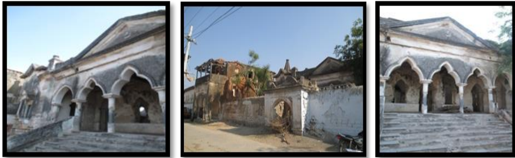
Fig.2.6: 101 entrance door (Nuttokka Darwaja) historical building Source: From field. Bhoodan Pochampalli, Oct, 2015.
