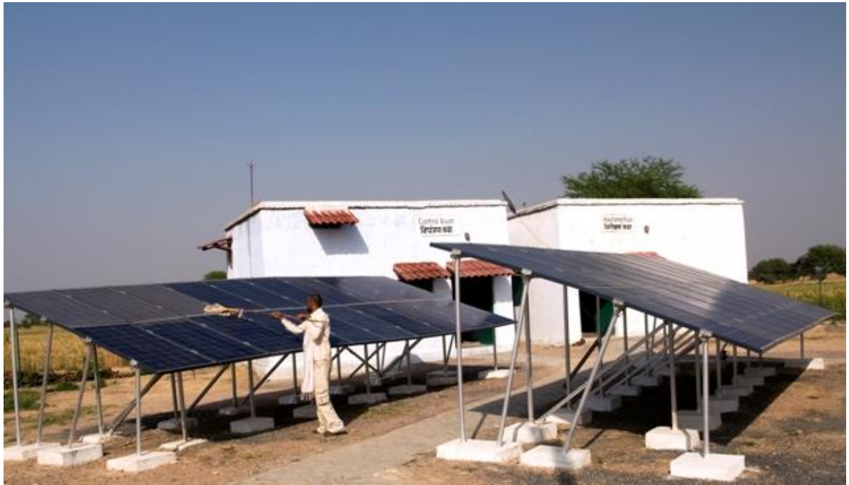
Note. Solar Panels of CSPP being cleaned manually by the villager in Rampura
