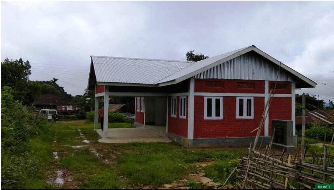
Image 3.2: Guest house constructed by Wildlife Trust of India
