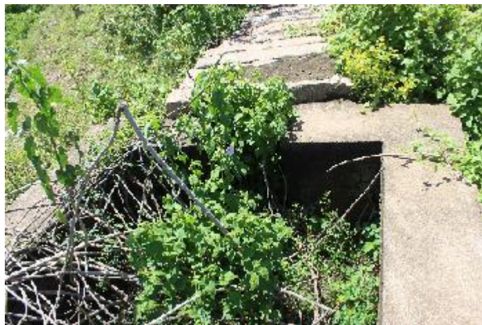
Plate 10, a closer view of the channel running
