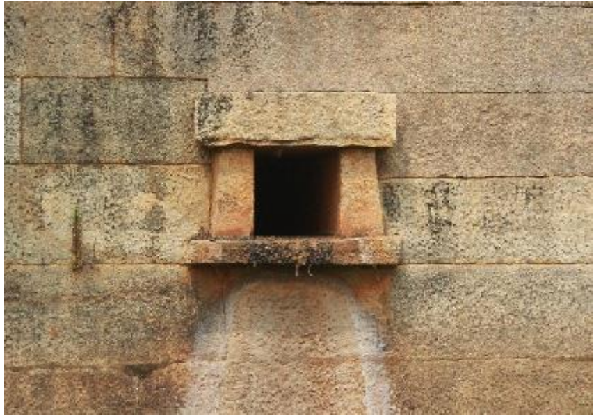
Plate 23, an inlet of the tank
