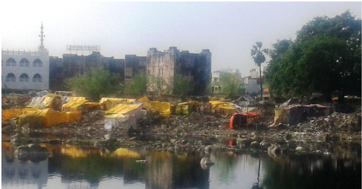
Picture 3. 4: Picture from Kotturpuram slum showing the poor housing condition of slums.
