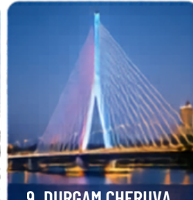
9. DURGAM CHERUVA CABLE BRIDGE
